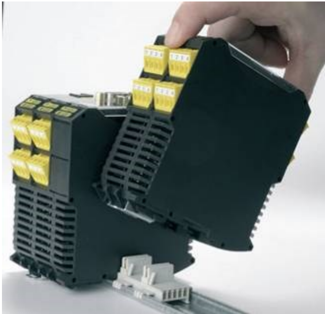
Fit module at an angle from above
